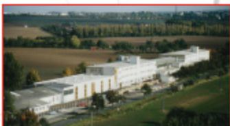
Rulmecca FAA GmbH Aschersleben, Germany
