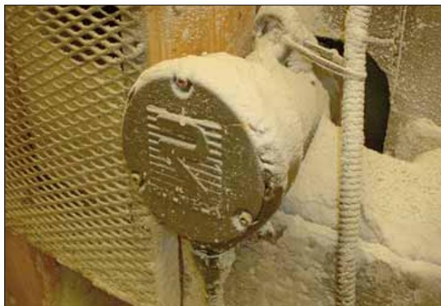
One of numerous Rulmeca Motorized Pulleys used by a major US salt producer, this 75 HP unit dramatically reduced maintenance expense while increasing conveyor drive reliability. The mine eliminated the need to grease external bearings and replace corroded drive components while reducing the oil change frequency to 50,000 operating hours by using synthetic oil. That equates to an oil change every six years.
