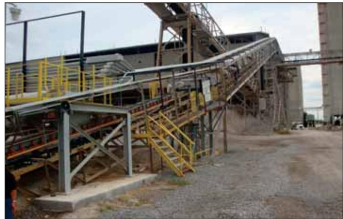
This US cement producer eliminated 4' of start-up belt bounce and subsequent belt and feeder damage on their concave reclaim tunnel conveyor when they upgraded from a 75 HP head pulley to two 50 HP Motorized Pulleys in the head and tail positions. The 360° of belt wrap decreased slack side tension and enabled the operator to use the existing belt in spite of the fact that installed power was increased by 33%.
