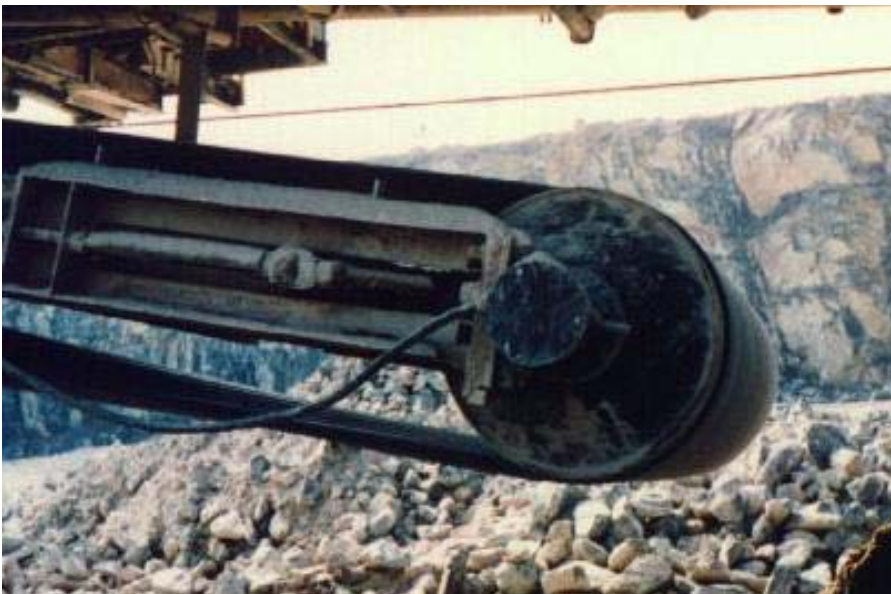
Fig. 15: Close-up of motorized pulley installed on TAKRAF mobile primary crusher in 1983. The motorized pulley concept simplified the mounting of this 50 HP conveyor drive in the tail position in a screw take-up.
