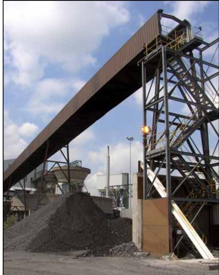
Figure 5 Kellingley Colliery replaced old problematic "bottom belt drive" near tail (left photo) on the main coarse discard conveyor in 2003 with 100 HP Rulmeca Motorized Pulley at discharge end above pile (right photo) and eliminated 300,000 tons of lost production annually.
