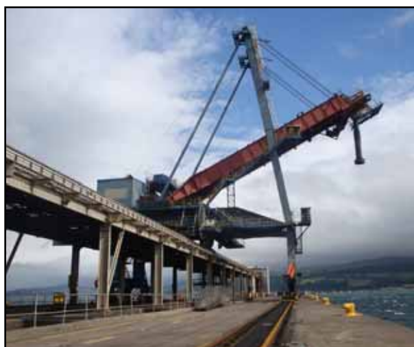
Figure 16 Model 1000HD will replace existing dock conveyor drive at this major Scottish coal export/import terminal in 2011.
