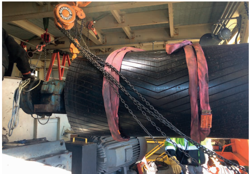
Figure 6. Live shaft pulley and two pillow blocks (above) and exposed motor and gearbox (below) during removal from service. Weight of original drive system was nearly 50% more than motorised pulley drive.
