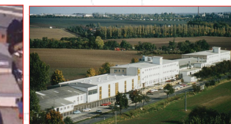
Rulmecca FAA GmbH Aschersleben, Germany
