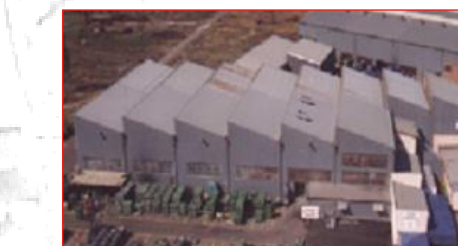
Melco Conveyor Equipment, Germiston, South Africa
