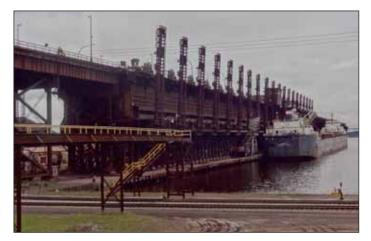
Since temperatures can reach -20° F at this iron ore terminal, night time frost can build up beneath the carrying strand of belt causing slippage at start-up. The installation of two 180 HP Motorized
