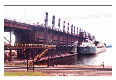
Since temperatures can reach -20° F at this iron ore terminal, night time frost can build up beneath the carrying strand of belt causing slippage at start-up. The installation of two 180
